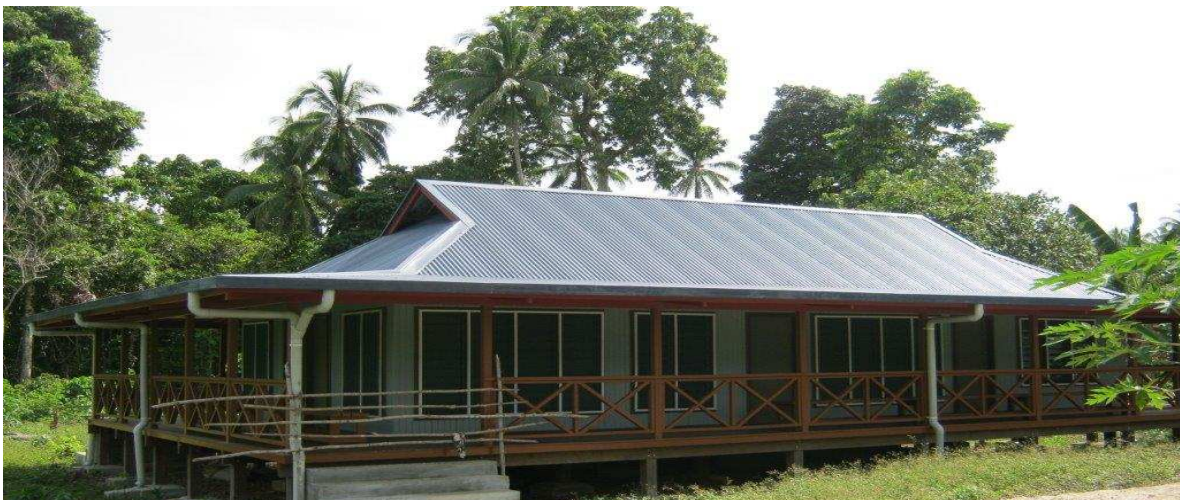
New aid post in Lau village, West Pomio, ENBP build with timber contributed by the community sawmill
